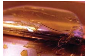
Major peel-off was observed.
